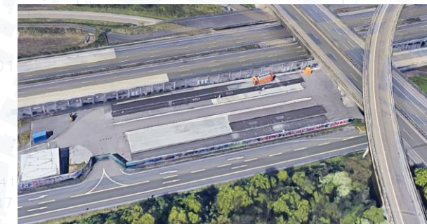
Полигон Federal Highway Research Institute (BASt), Германия
